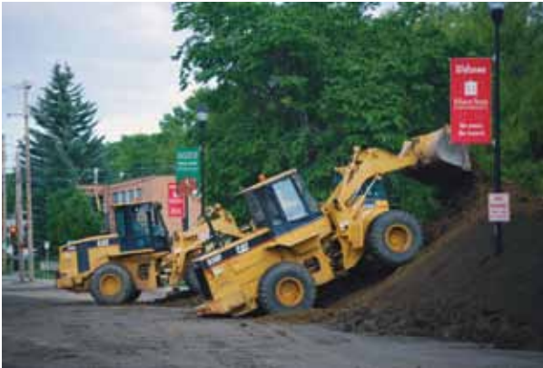
Construction crews work tirelessly to complete the "Beaver Dam."
